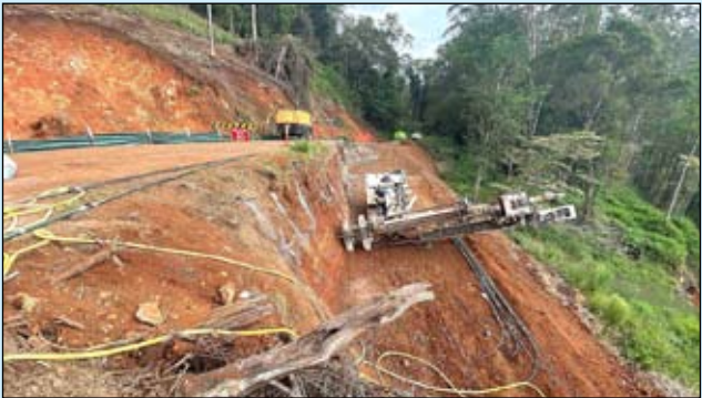
Tuntable Creek Road restoration included work performed by a 16-tonne hydraulic crawler mounted drill rig. This remote-operated machine is designed for safe access to undertake geotechnical restoration works, and is drilling around 8m into the embankment.
