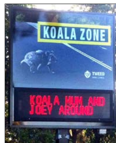
One of the variable message electronic signs and pavement treatment installed on Clothiers Creek Road, to raise awareness about the benefit for both koalas and road users of keeping to the speed limit.
