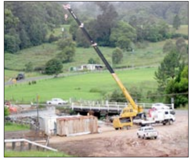
Bridgework. Work is progressing well on all the bridge replacements being undertaken throughout the region, despite delays caused by rain and holidays. Above: Mount Burrell.
