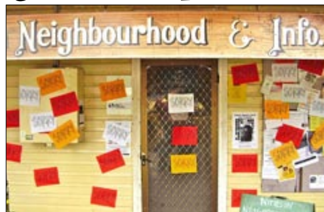
Sorry sight. The newly-renovated NNIC building, festooned with Sorry signs on 13th February. Photo: Natalie Meyer
