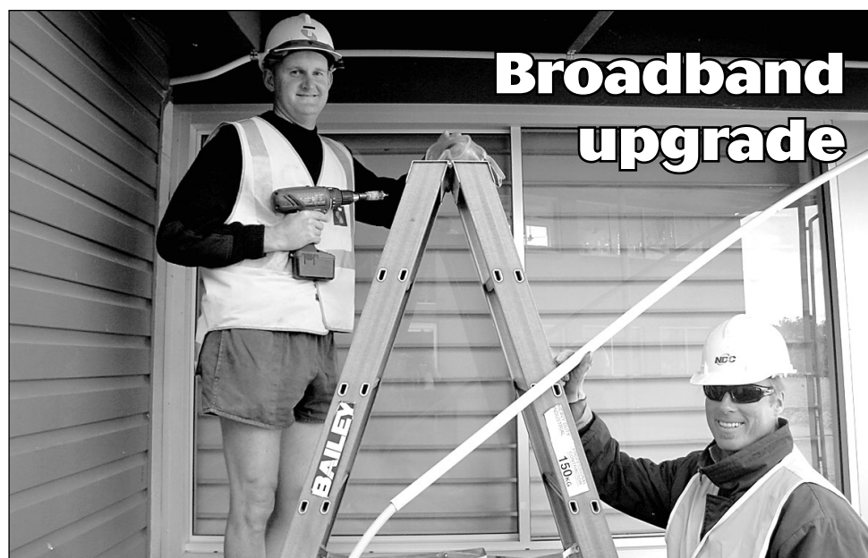
Wired. Adam Leonard and Rod Mitchell from Telstra installing new optical fibre broadband service at Nimbin Central School. Photo: Sue Stock
